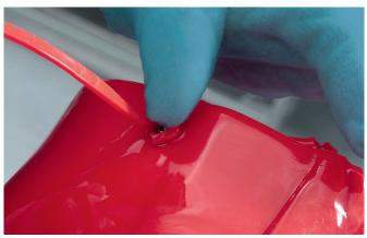
**TIP:** Infilling is only required if the lamination disk is not covered sufficiently.
